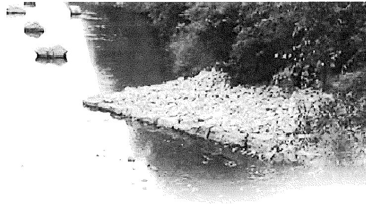
Figure 18. Deflector. These deflectors can be built alongside the river or stream to proactively direct the direction of the waterflow as well as create side coverage for brook trout (Lutz, 2007).
